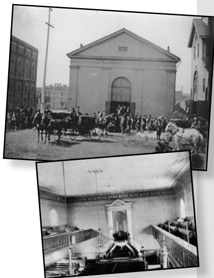
Grace Lutheran Church in downtown Milwaukee was constructed in 1851. Incorporated in 1849, Grace was where three Lutheran pastors met to discuss founding a synod that would eventually be known as WELS.
