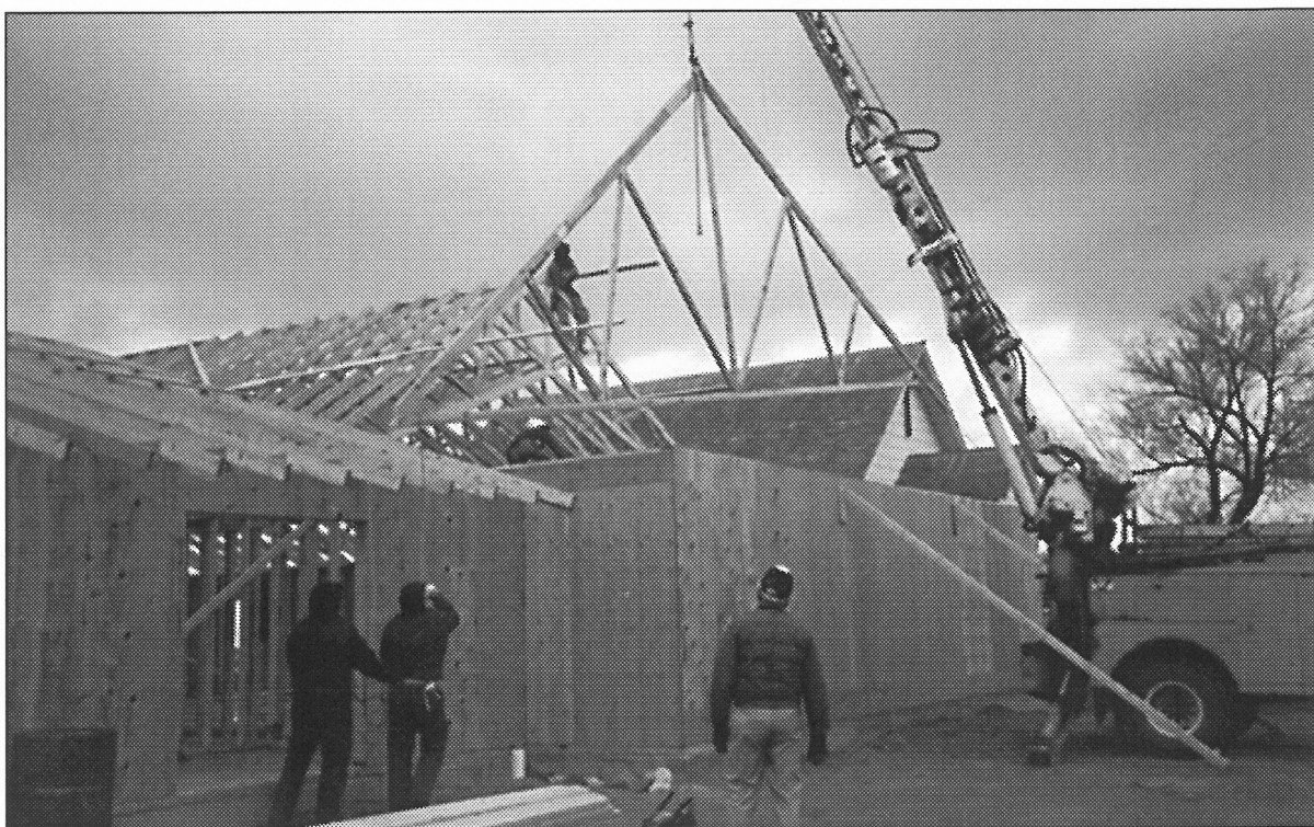
Volunteers and workmen are making progress on the building of the new Lutheran Church in Martin. According to Ken Boomer, the structure could be enclosed within the next few weeks. The top photo was taken Monday, May 7, 1990 and the bottom photo was taken this morning, Wednesday, May 9, 1990.
