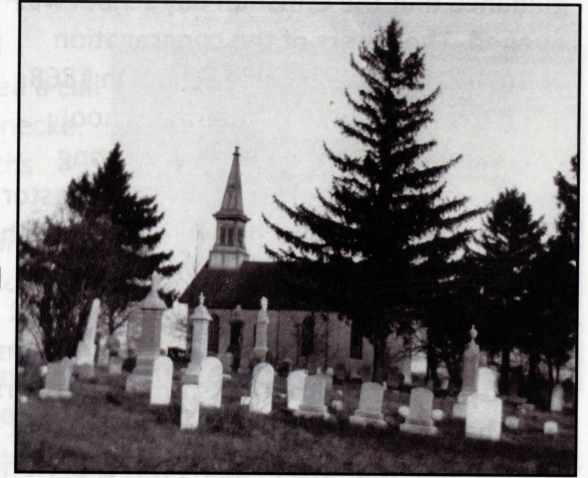
1863 church with original steeple
