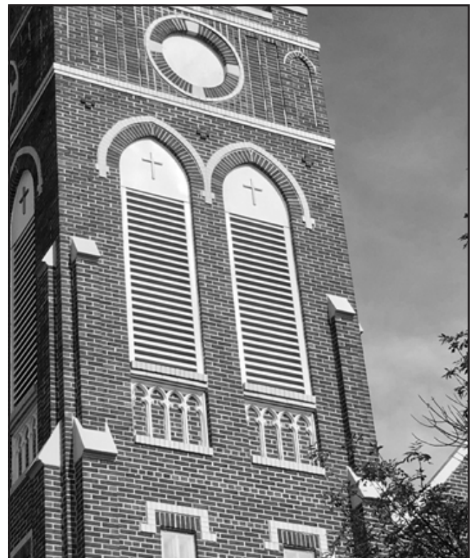
New louvers were installed on the bell tower in 2017.
